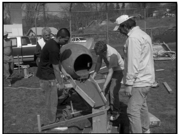
Foundation work begins. Photo by Mildred Lykens
